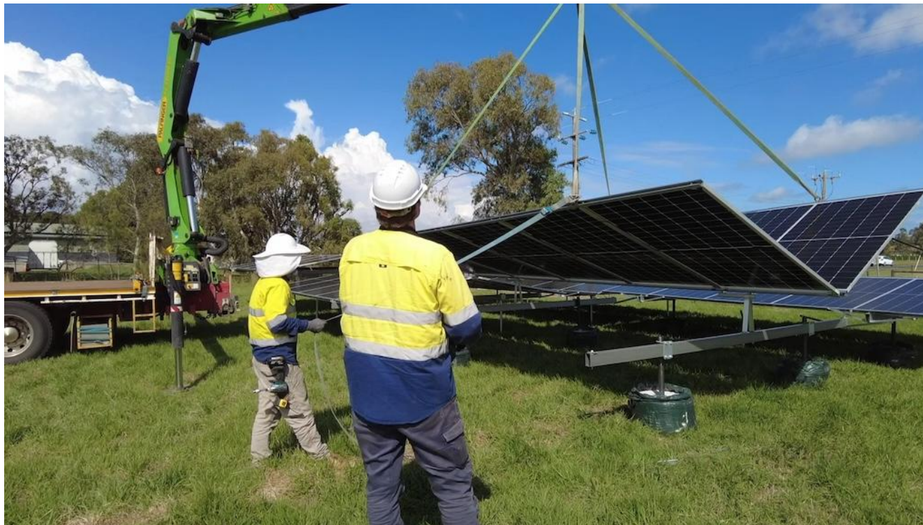
Solpod being unfolded onto a ground frame
