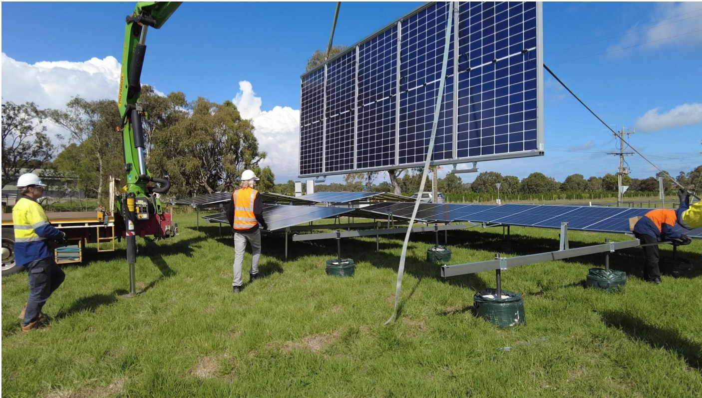
Using a crane to lift a Solpod onto a ground frame
