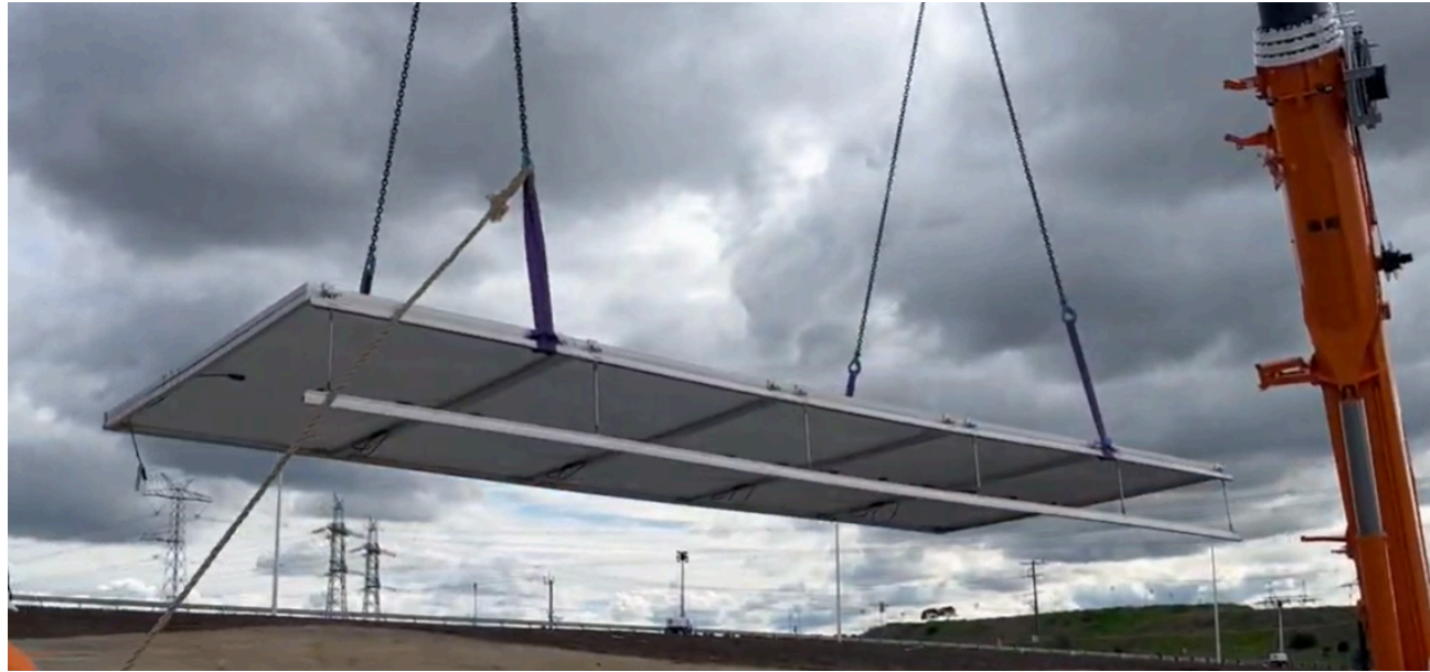
Solpod being lifted in a horizontal orientation
