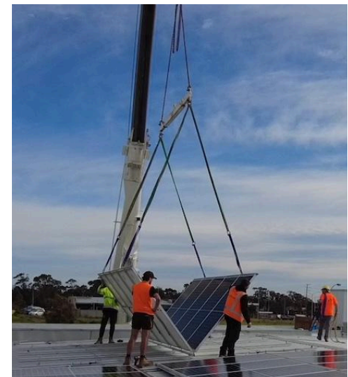
Solpod being unfolded on roof
