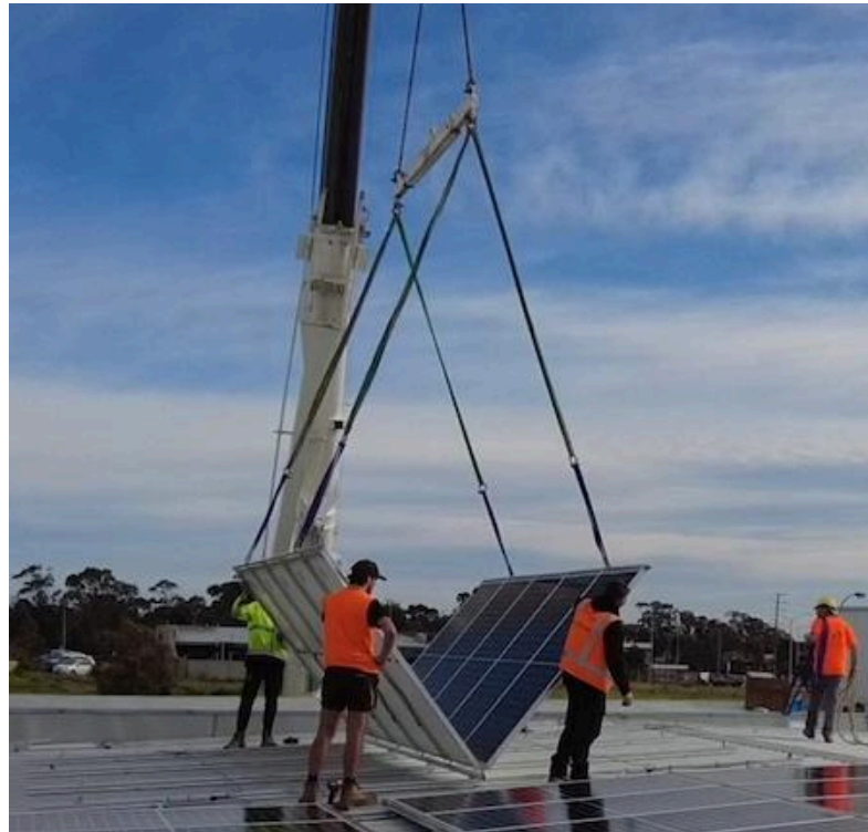
Solpod being unfolded
