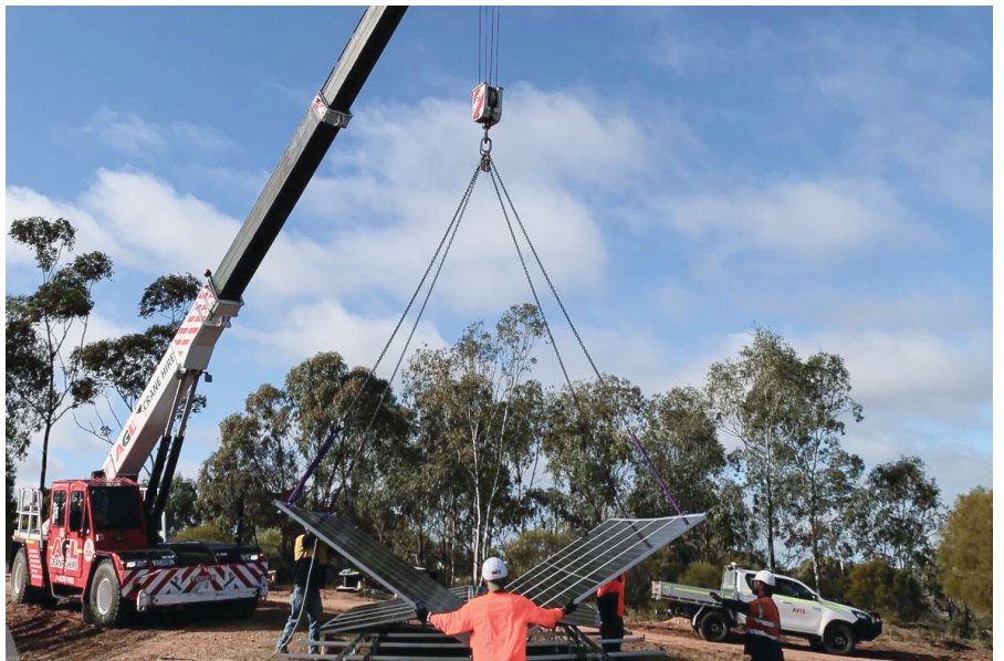
Crane unfolding a pod onto a subframe
